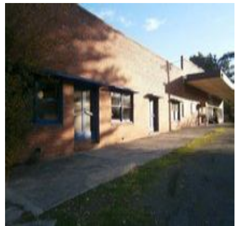
The former Kongwak post office and general store.
