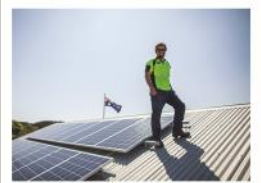
6.0Kw System, Inverloch RSL
