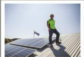
6.0Kw System, Inverloch RSL
