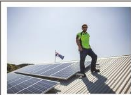
6.0Kw System, Inverloch RSL
