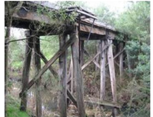
Lang Lang River Bridge. Photo: Heritage Council Victoria
