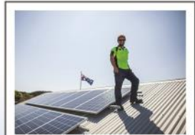
6.0Kw System, Inverloch RSL
